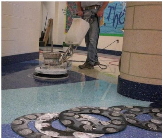
This system can be used with conventional cleaning/maintenance equipment such as auto scrubbers, electrical or propane burnisher, swing machine, buffer, etc. for restoration – grinding and polishing of natural stone, terrazzo, and concrete floors
